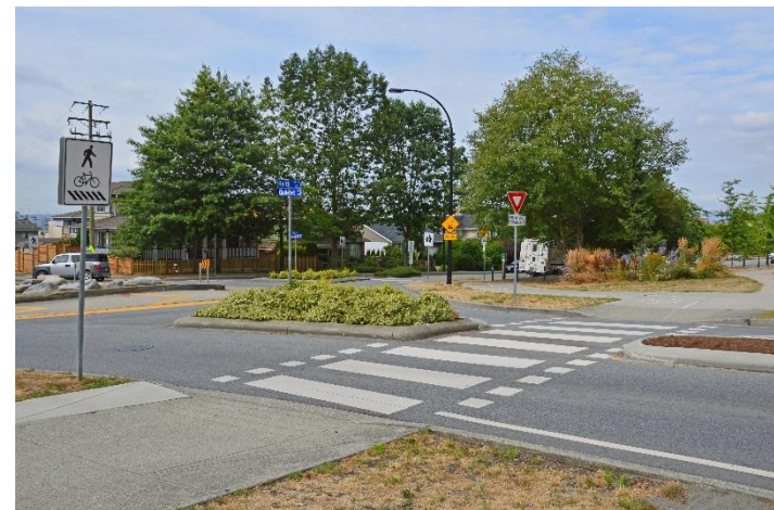
Combined crosswalk and cross-ride on the Spirit Trail in North Vancouver, B.C.
